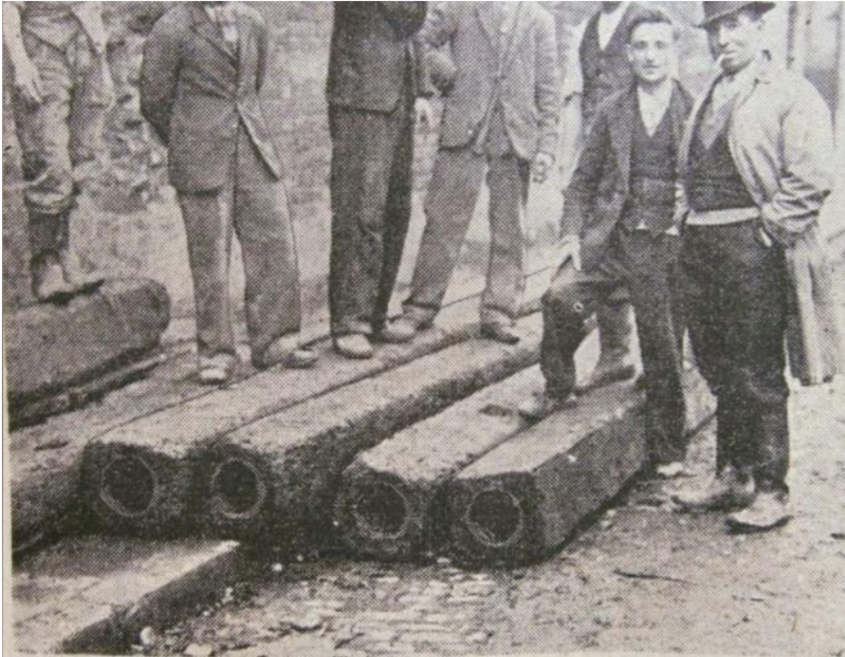
Workmen photographed with some of the old wooden water pipes which were unearthed at Marrowbone Lane during the housing scheme excavations. They were laid by the Huguenots about 250 years ago.
